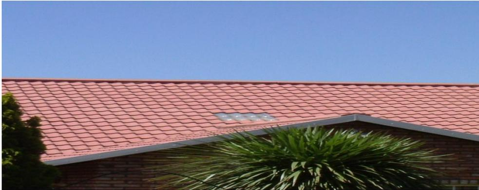
***2MM THICK, VACUUM FORMED POLYCARBONATE TRANSLUCENT TILE***
